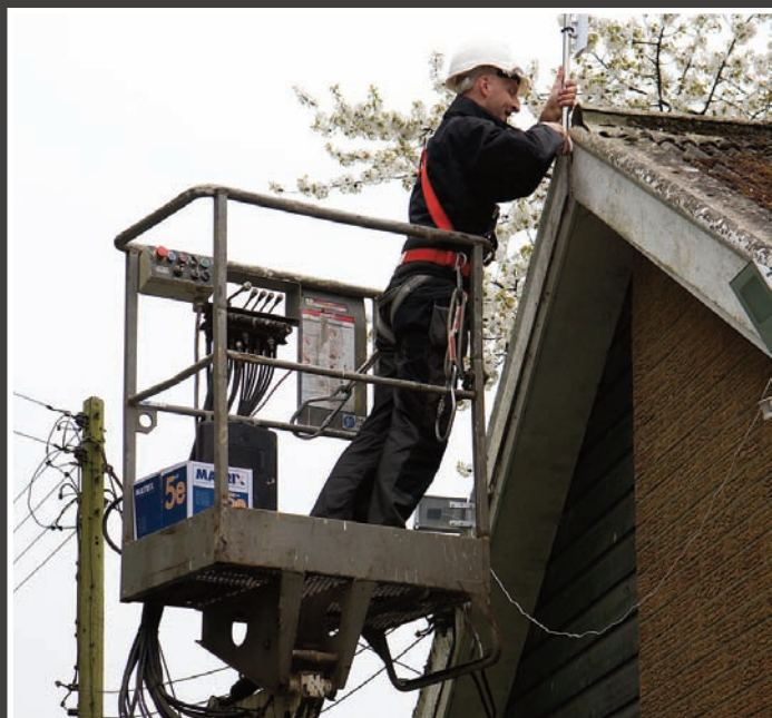
Broadband being installed
