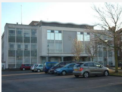
Old Guildhall redevelopment site.
