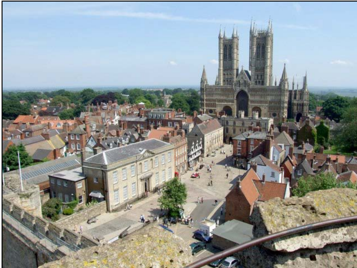
The Proposed Scheme will be only visible from the very top of Lincoln Castle Tower.
