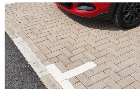
PCC block paving - parking bays
