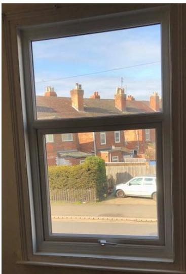
**Background:** The windows to the property were found to have rotten wooden frames with single glazing, and were causing damp and mould and poor thermal efficiency. An improvement notice was served and the new windows were fitted throughout the property.
