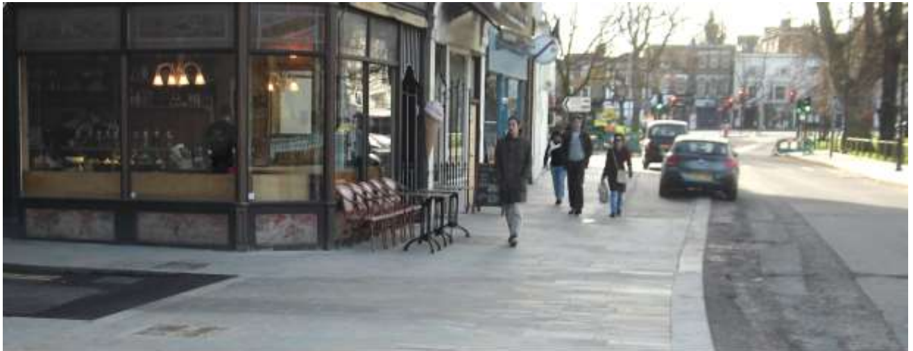
Figure 7-8 - Continuous Footway (Bromells Road, Clapham) (Source: CIHT Designing for Walking, 2015)
