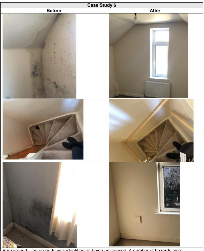
Background: The property was identified as being unlicensed. A number of hazards were assessed including extensive damp and mould throughout the property and a lack of handrails on staircases. An improvement notice was served to require works to be carried out.
