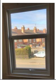
**Background:** The windows to the property were found to have rotten wooden frames with single glazing, and were causing damp and mould and poor thermal efficiency. An improvement notice was served and the new windows were fitted throughout the property.
