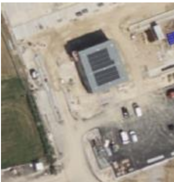
Figure 11-2 Caenby Corner Depot, showing roof mounted solar PV array
