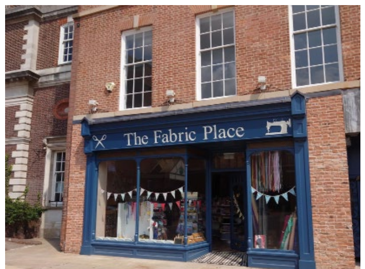
THI Gainsborough Market Place
